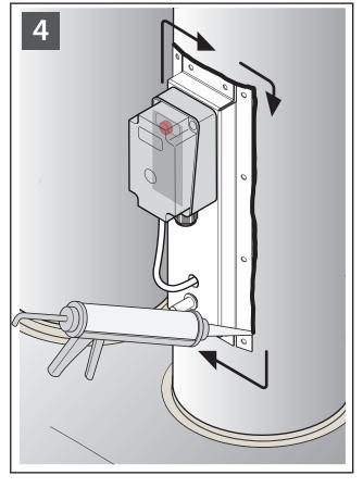
3 Installation of frost switch
